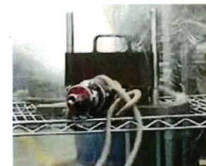
SOME RUBBER LINED HOSE IS COMPROMISED
