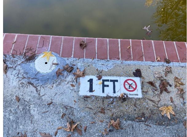
Figure 56 Repaired Skimmer Area
