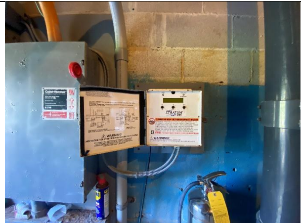
Figure 52 Vacuum Release System
