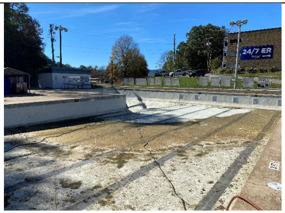
Figure 4 Swimming Pool (NE Corner)
