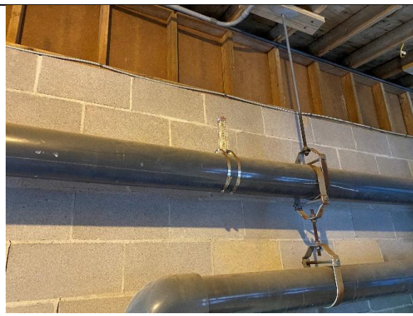
Figure 48 Pool Flow Meter
