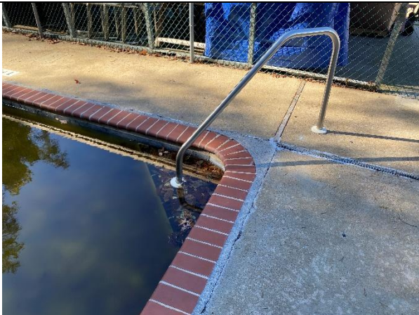
Figure 57 Stair Entry Railing
